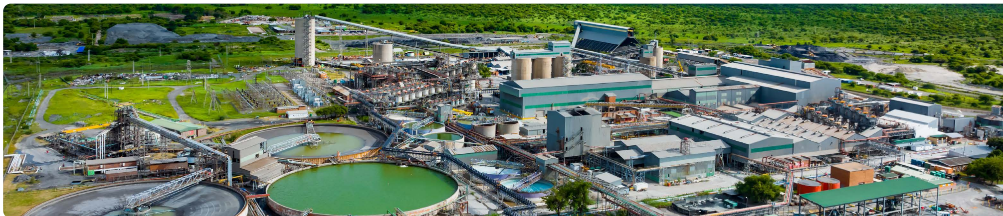
Aerial view of the Amandelbult chrome plant
