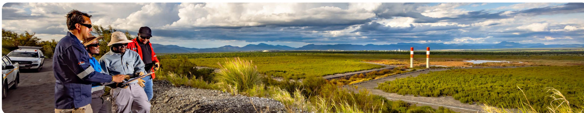
Overview of the tailings storage facility at Amandelbult
