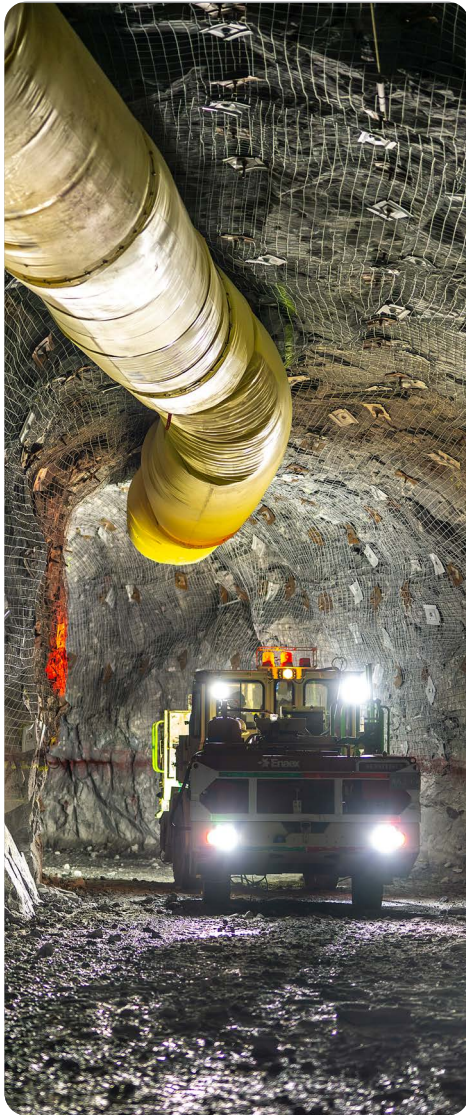
Charging unit travelling through tunnel at Mogalakwena
