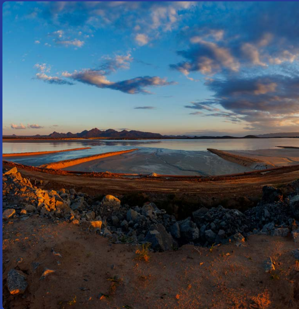
Mogalakwena's Blinkwater tailings storage facility
