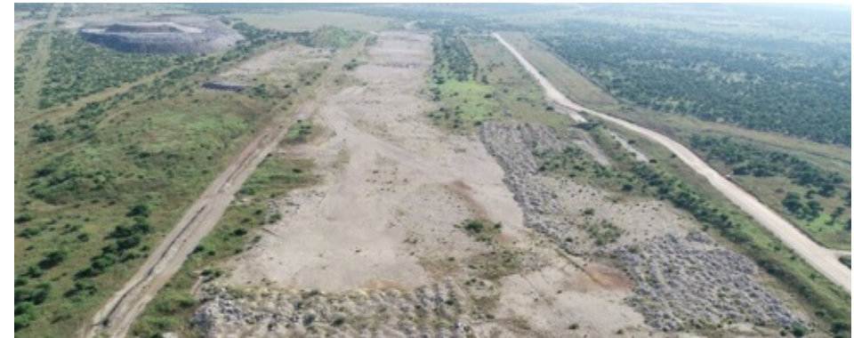
Pit 4&13A before backfilling
