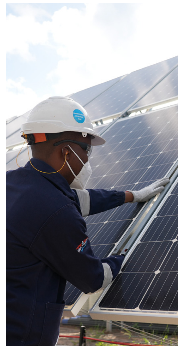
James Kutumela , general assistant , inspecting the solar PV panels at Mogalakwena Mine
