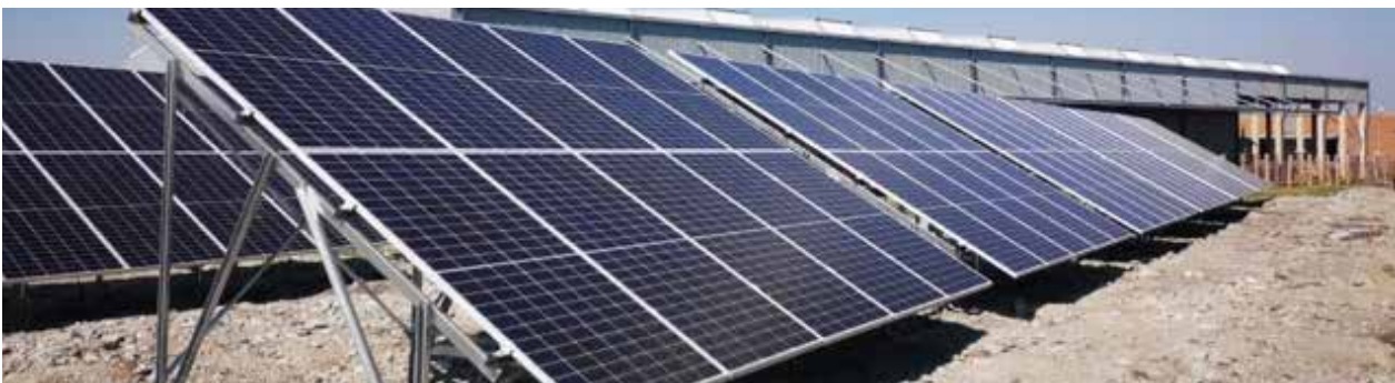
Western Limb Distribution Centre 350kWp fixed-axis ground-mounted solar PV plant.
