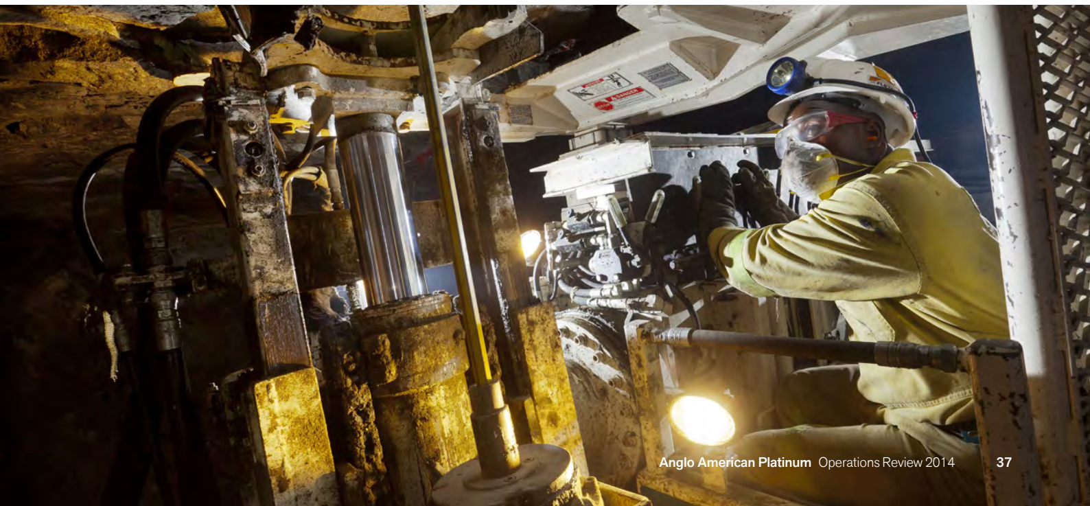
Roof bolting, Unki Mine
