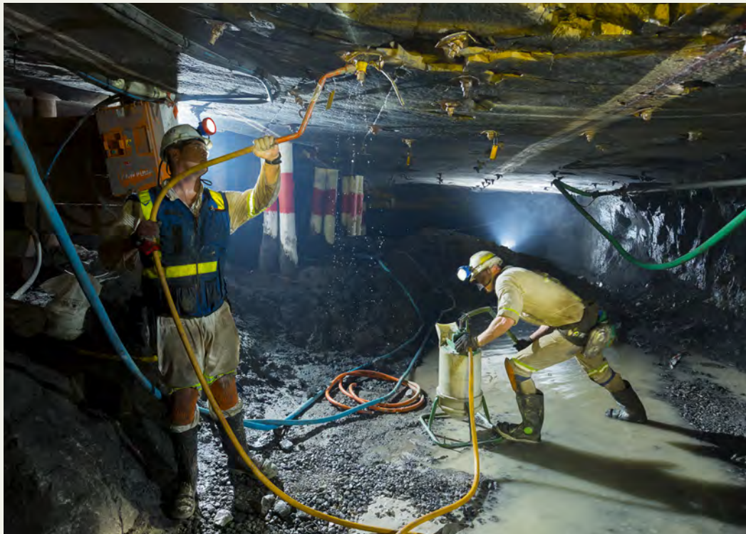
Installation of a flexibolt at Bathopele Mine.
