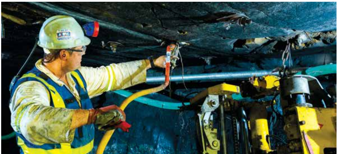
Image Installing a flexibolt at Bathopele Mine.
