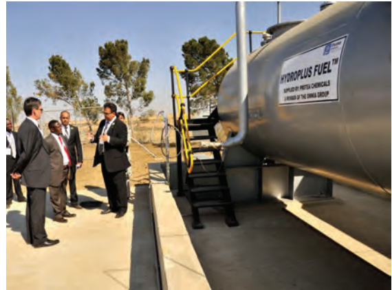
Opening of the world's first Rural Fuel Cell Mini grid, to power the Naledi Trust community - 5 August 2014
