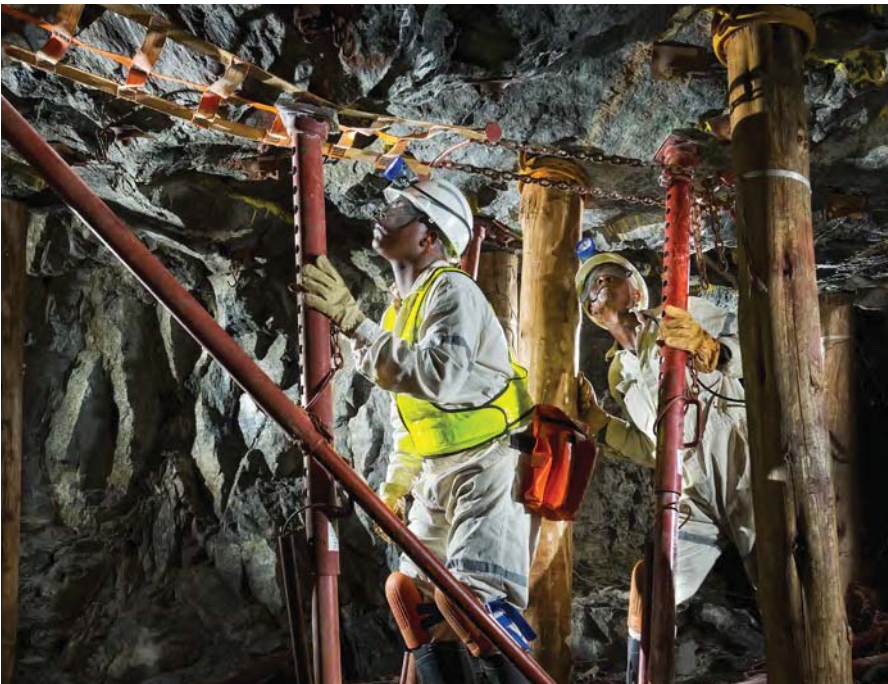
01 Lucas Mathe and Lefa Sedumedi installing and inspecting canopy jacks to secure a brow.
