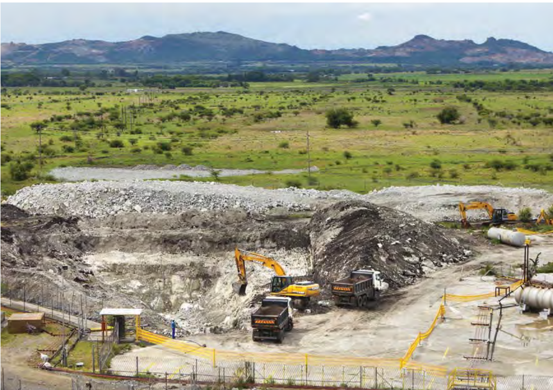
Pandora chairlift decline shaft being excavated.
