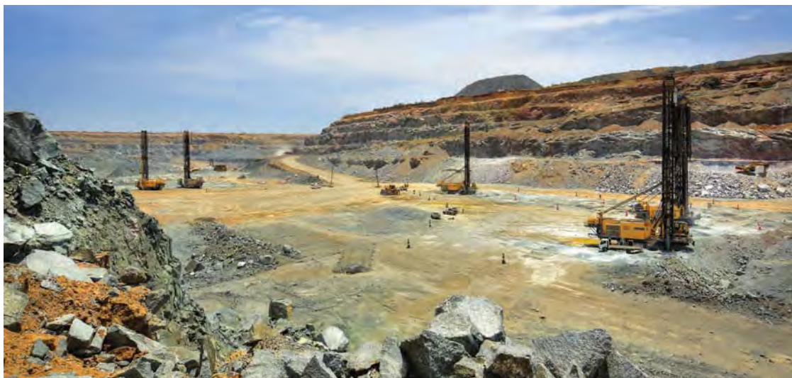
01 Pit viper drill rigs in operation at Mogalakwena North Pit 02 Bheki Mhlanga, Engineer section surveyor, surveying the North pit at Mogalakwena Mine.
