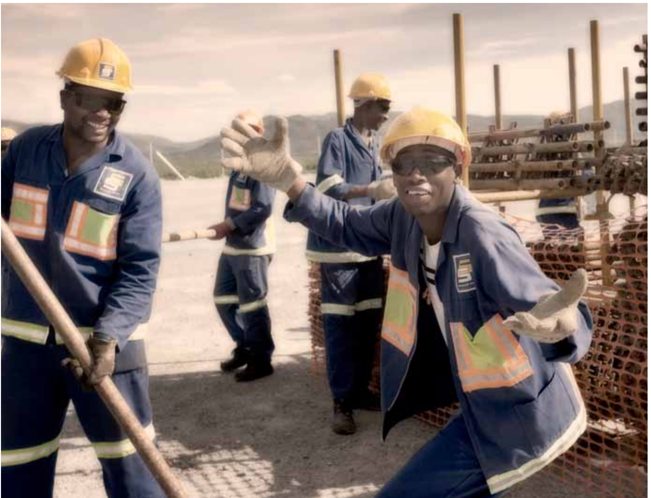
Construction workers at Styldrift
