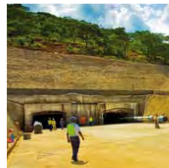
Development work at the Unki project progressed steadily in 2006
