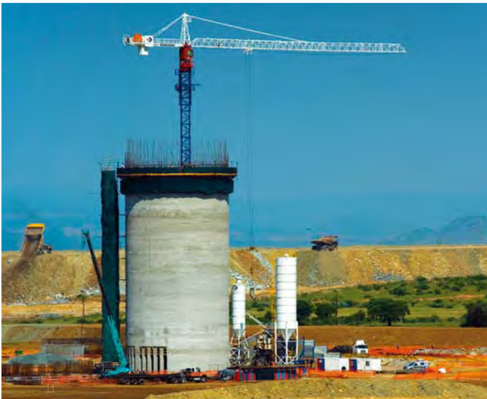
Construction work on the new PPRust concentrator
