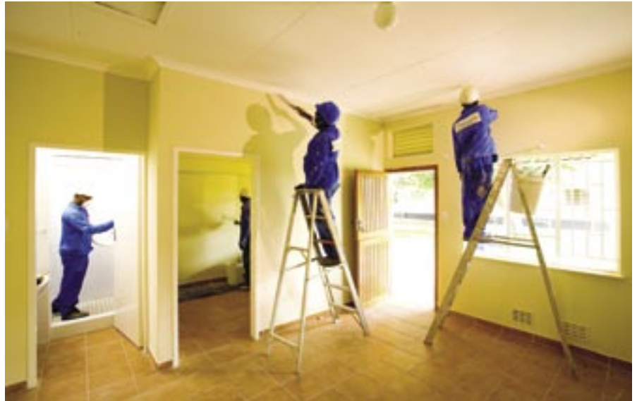
Contractors applying the finishing touches to an apartment for married couples at Jabula Hostel near Townlands Shaft at Rustenburg Section.
