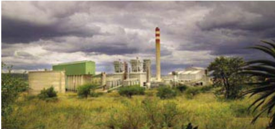
Polokwane Smelter, located in Limpopo Province
