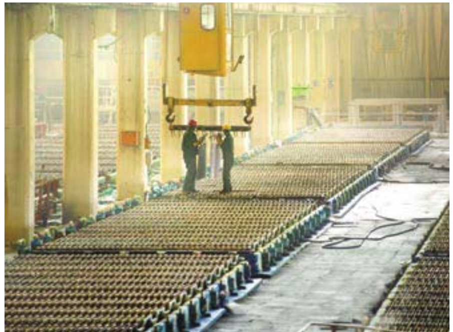
The tankhouse at RBMR where nickel and copper cathodes are produced.
