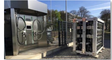
Performed high speed hydrogen refuelling tests and hydrogen storage installed .
