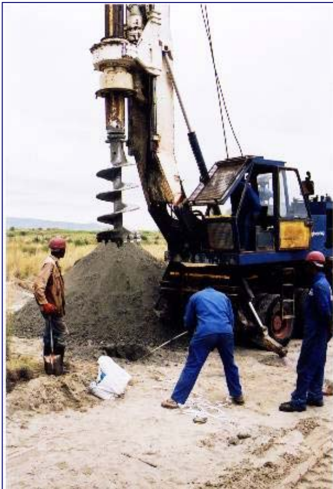
Large bore auger drilling
