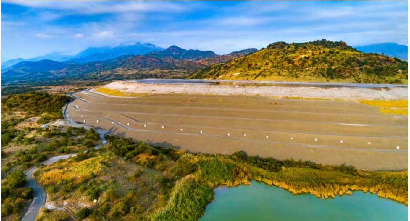
Work was done on the reinforcement of the Helena tailings dam
