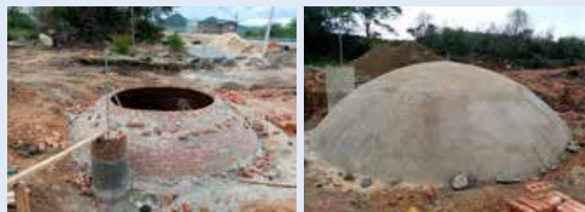
Construction of Unki's biodigester
