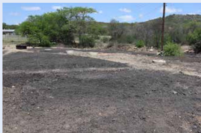
Levelled area after construction was completed
