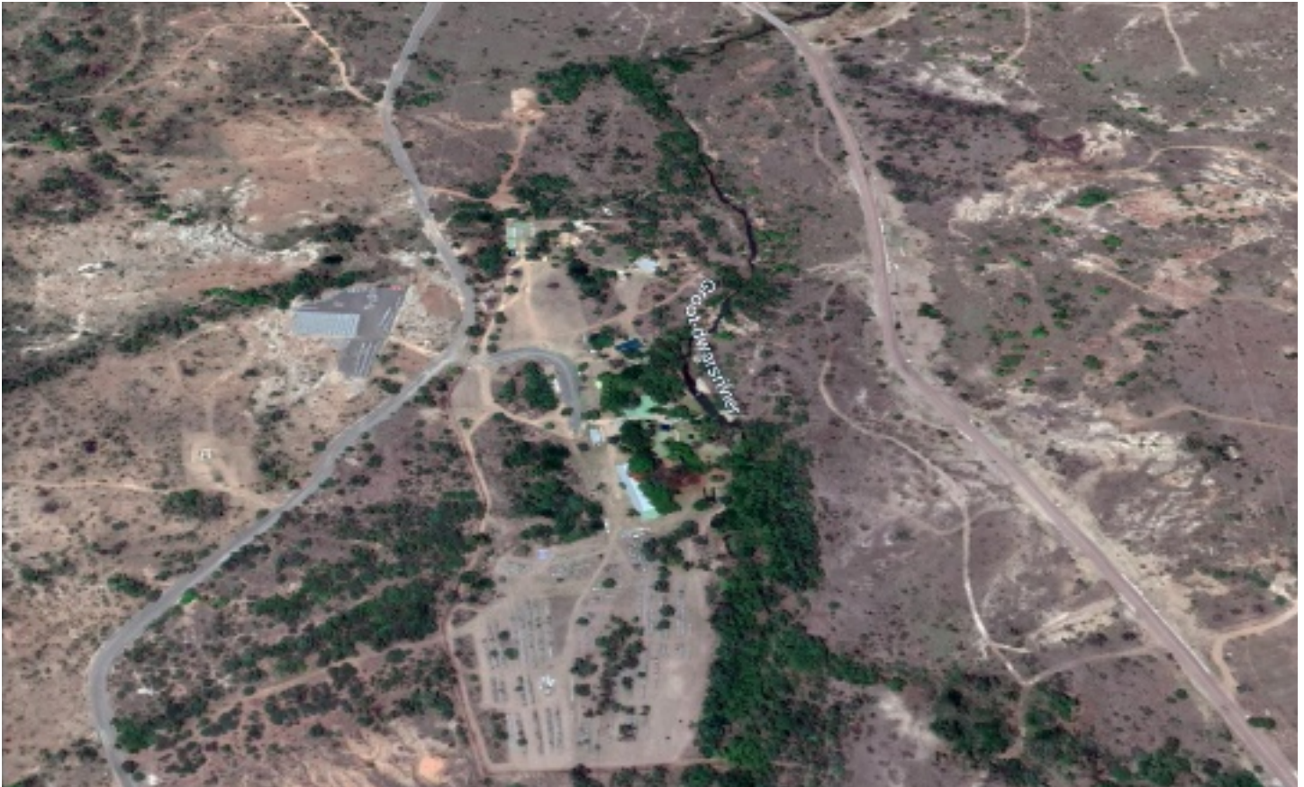
Figure 5: A bird's view of Mototolo Der Brochen Mine Complex. Source: Anglo American (Der Brochen Amendment Draft Scoping Report), 2019
