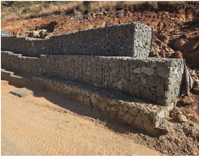
Photo 13: Drift 1 - gabions, geotextile and reno mattresses
