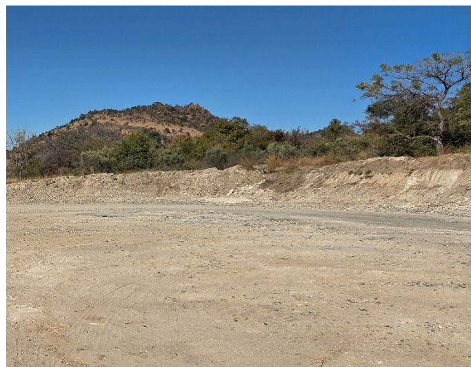
Photo 10: Borrow Pit 1 - erosion gullies along the stockpiles
