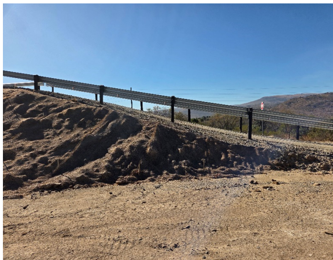
Photo 20: Borrow Pit 1 - Enviromat® along the brake test ramp as part of ongoing rehabilitation
