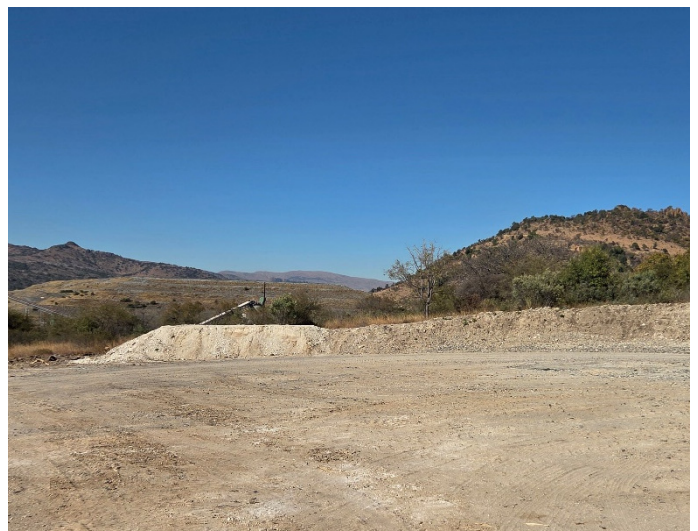
Photo 18: Borrow Pit 1 - berms at the topsoil stockpiles
