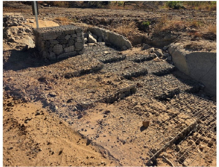
Photo 14: Drift 5 - gabions, geotextile and reno mattresses
