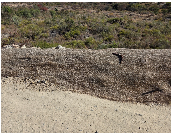
Photo 17: Access route 1 - cut-off berm with Enviromat® installed as part of rehabilitation
