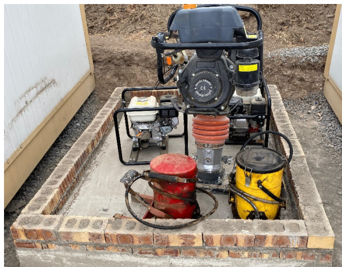
Photo 6: Concrete bunded area for equipment
