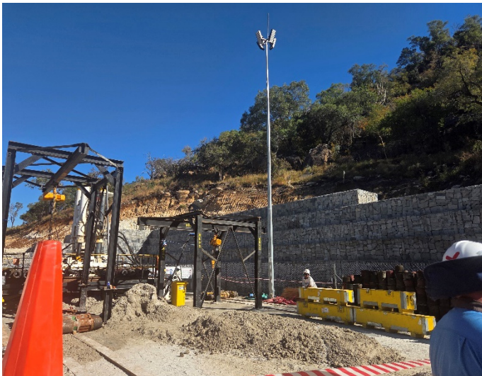
Photo 15: Borwa Downcast South Vent Shaft construction site - upgradient gabions
