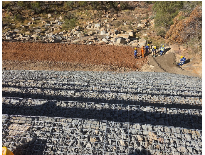
Photo 16: Borwa Downcast South Vent Shaft construction site - downgradient gabions
