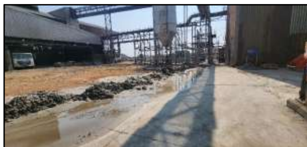
Picture 10: Water flowing in plant
