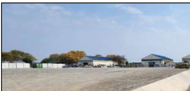
Picture 27: Roof structure painted
