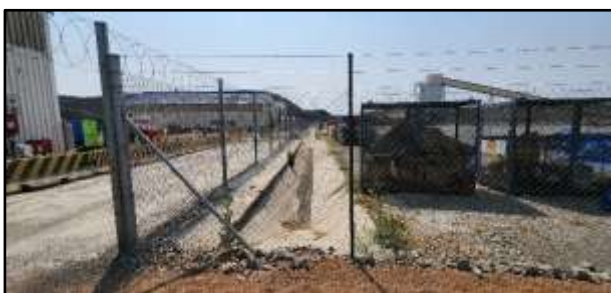
Picture 37: SO 2 facility fencing.
