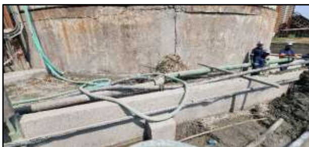
Picture 9: Sedimented bund in the process of cleared
