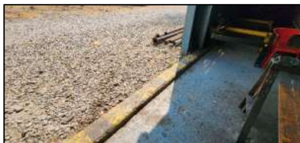
Picture 34: Workshops fitted with clean and dirty water separation
