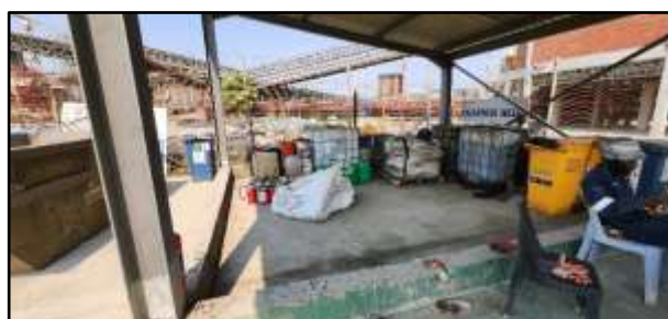
Picture 16: Bunded hazardous waste storage
