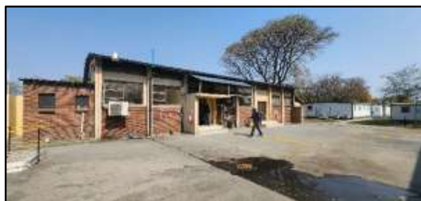
Picture 26: Buildings painted in non-reflective, natural colours.
