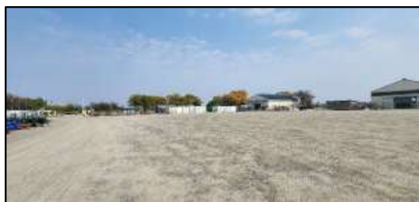
Picture 38: Cemented stabilised surface of the SO 2 facility construction area.
