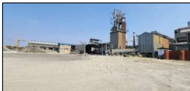
Picture 28: Infrastructure painted
