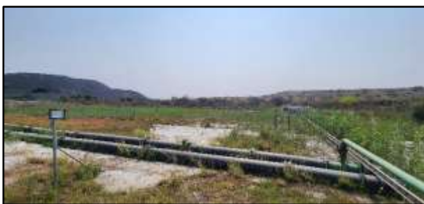
Picture 21: Site fencing
