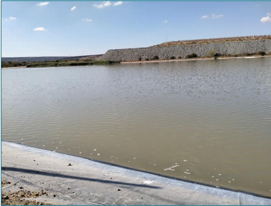
Figure 3.4-5: Return water dam
