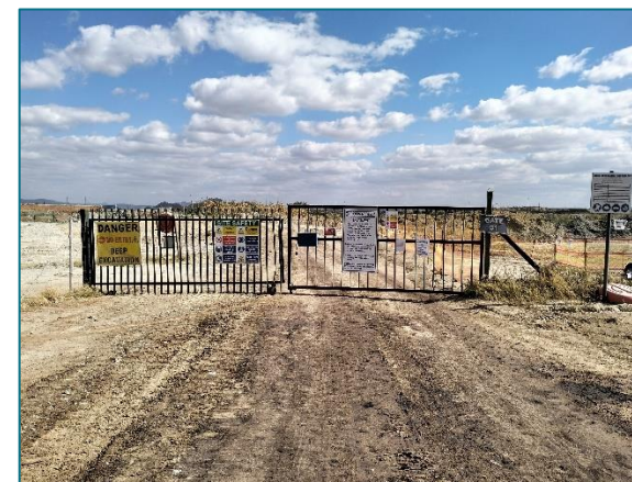
Figure 4.2.1-4: PCD fence and signage
