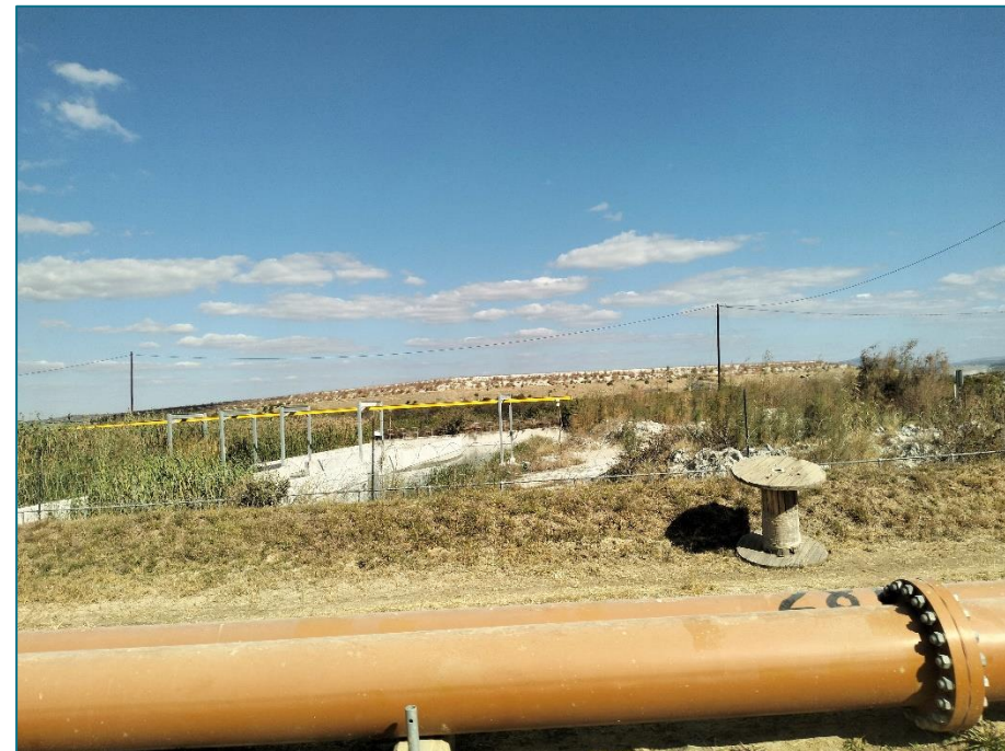
Figure 3.4-2: Blinkwater TSF sump
